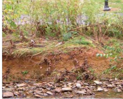
A moderately stable streambank has some vegetation and may or may not have a vertical bank.
