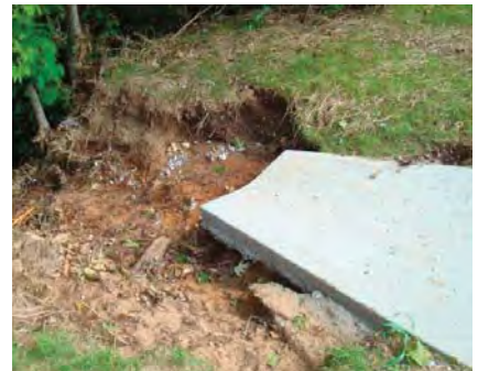
Runoff delivered to a creek by level spreader with no riprap protection or vegetative filter strip will deliver pollutants and become an erosion problem before entering a stream.
