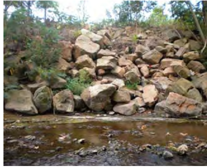
Riprap is an unsightly form of streambank protection that offers no pollutant filtration, wildlife habitat or aesthetics but can fix an unstable bank.
