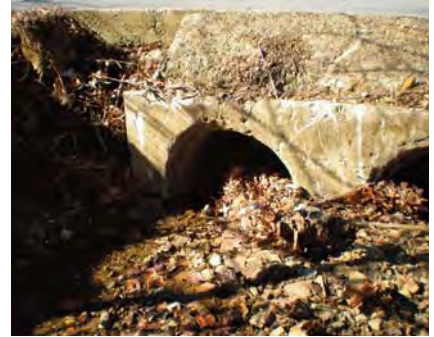
Culverts can clog with woody debris, trash and sediment. When this occurs, water flow can be blocked and aquatic wildlife movement can be limited.
