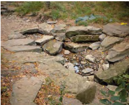
A cross vane rock structure incorporated with vegetation as part of a natural channel redesign will not likely have to be replaced.
