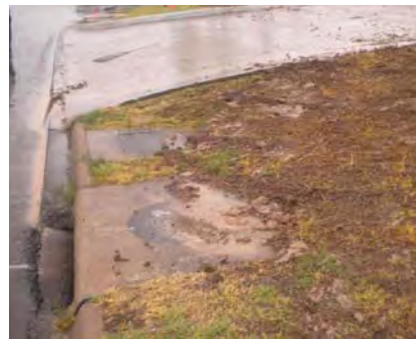
Sediment in streams can come from many places, but often the source can be found with simple investigation.
