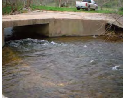
Low-water bridges installed without proper design can often block or limit both water flow and aquatic life movement up and down stream.
