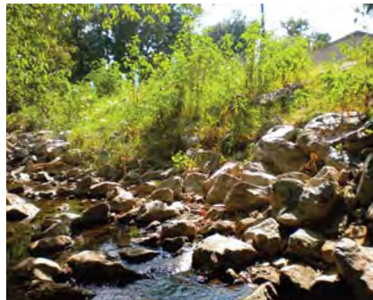
Riprap placed at the bottom of a re-sloped bank with vegetation added for increased beauty and strength will not likely have to be replaced.
