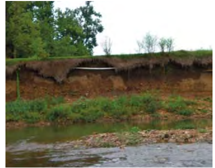
A streambank stripped of its natural protective vegetation and without any type of restoration is completely unprotected and highly erosive.
