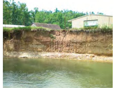
A highly unstable streambank has little to no vegetation and a vertical bank.
