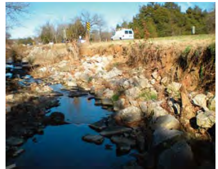
Riprap placed at the bottom of a vertical bank with no re-sloping or vegetation added will likely have to be replaced.
